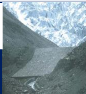
Outlet channel with reinforced dam reconstruction at the moraine dammed lake Laguna Cuchillacocha, Peru
