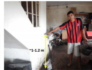
Fig. 9. A residential house showing the estimated peak height to be 1 to 1.2 meters.
