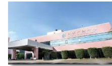
I&T Facility Completion
