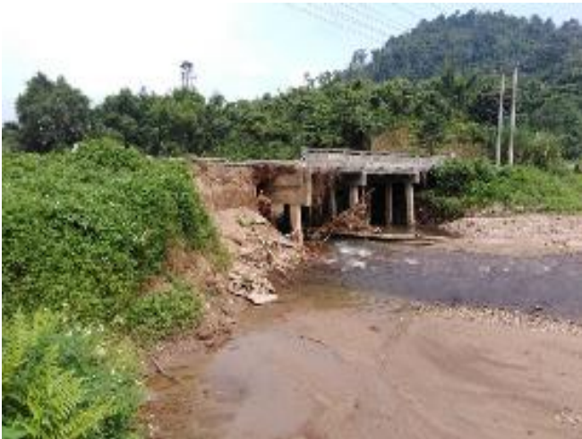
Bridge on R3 (Photo on 6 October 2018)
