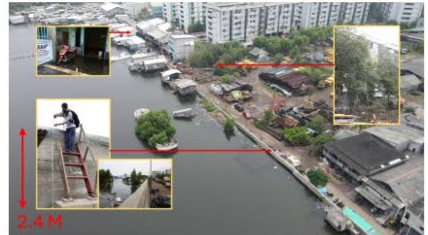
Muara Baru Jakarta 2.4 meters under the sea level (Widodo, 2024)
